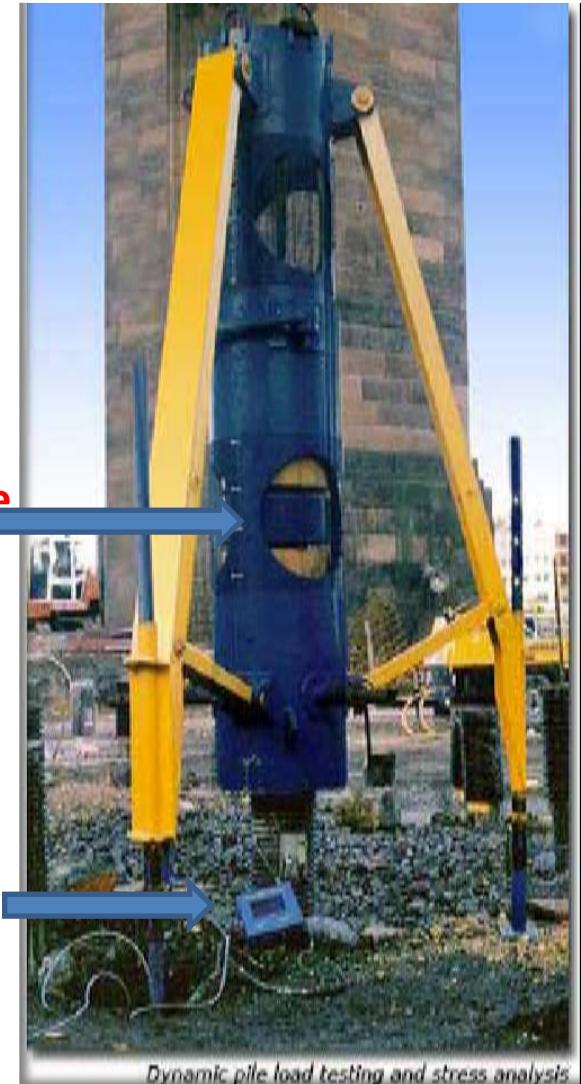
Dynamic pile load testing and stress analysis
